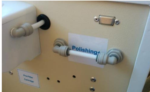
Figure 33. Inserted bypass tube.
